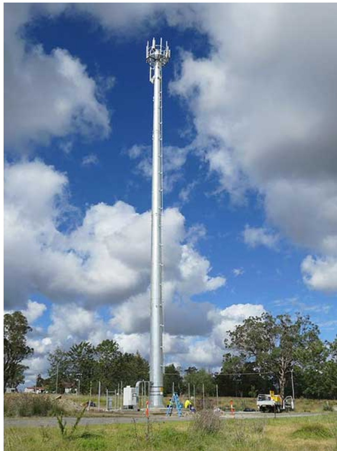
Typical 30 metre tall NBN wireless internet tower.
